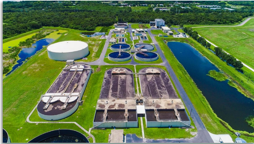
Wastewater Treatment Plant Source: Manatee County
