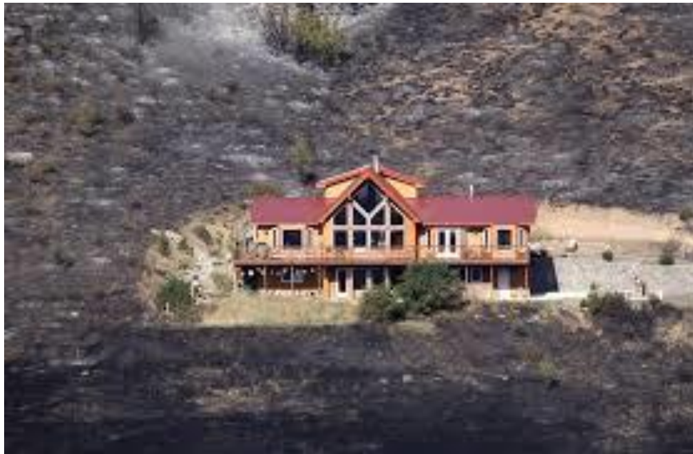
The photo above demonstrates how defensible space guidelines can help save a structure from wildfires.
